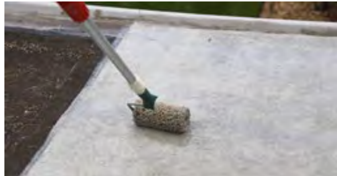
Two people are required for laminating the roof. One to apply the basecoat with a soft roller and another to consolidate with a paddle roller.
