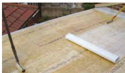
A polyester roller is used to apply the resin to the Reinforcement Mat. Cure It Roofing Resin is applied to the deck before the Reinforcement Mat is laid on the roof.
