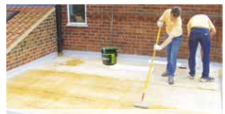
After the Reinforcement Mat has 'wet out', the consolidator roller is used to expel air from the laminate and ensure the Reinforcement Mat has been saturated by the resin. No white patches should be visible. As the Reinforcement Mat absorbs the resin, the laminate becomes transparent.
