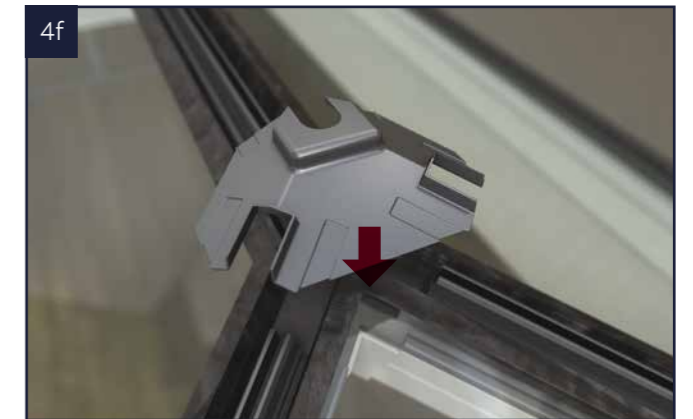
Position the ridge end seal in place ensuring it is central to the hip bars and ridge.
