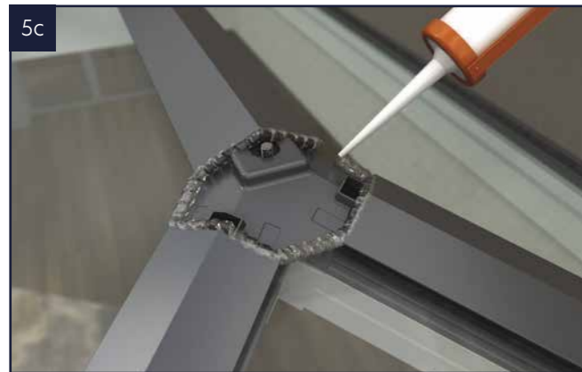
5c Apply sealant to the top of the ridge end seal.
