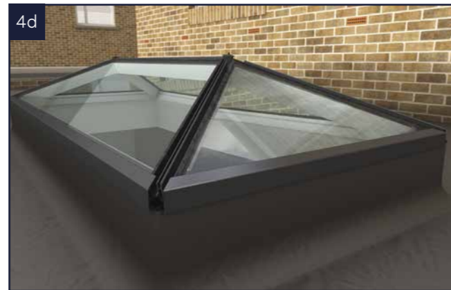
Position all four glass sections ensuring they are central to the lantern assembly with equal spacings either side of the hip bar.
