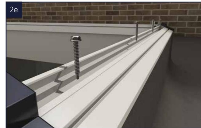
2e Fully fix down the entire ringbeam around the perimeter at approximately 100 mm from each corner and 400 mm centres using LRSB001 A2 Stainless hex head tech screw (4.8 mm x 50 mm).
