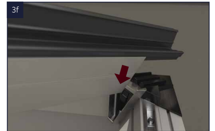
3f Ensure all the hips line up with the ringbeam corners. With a downward motion click the hips into place. Check all hips are locked into place at all four corners by applying an upward force on the hip.
