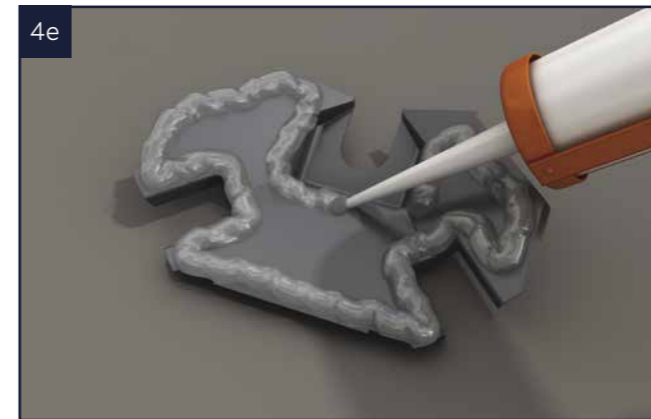
Apply sealant to the underside of the ridge end seal.
